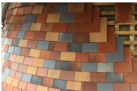
Clay tile façade assembly
