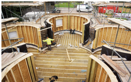
Assembly of ground floor timber frame
